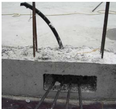
Post Tensioned Concrete Slab
